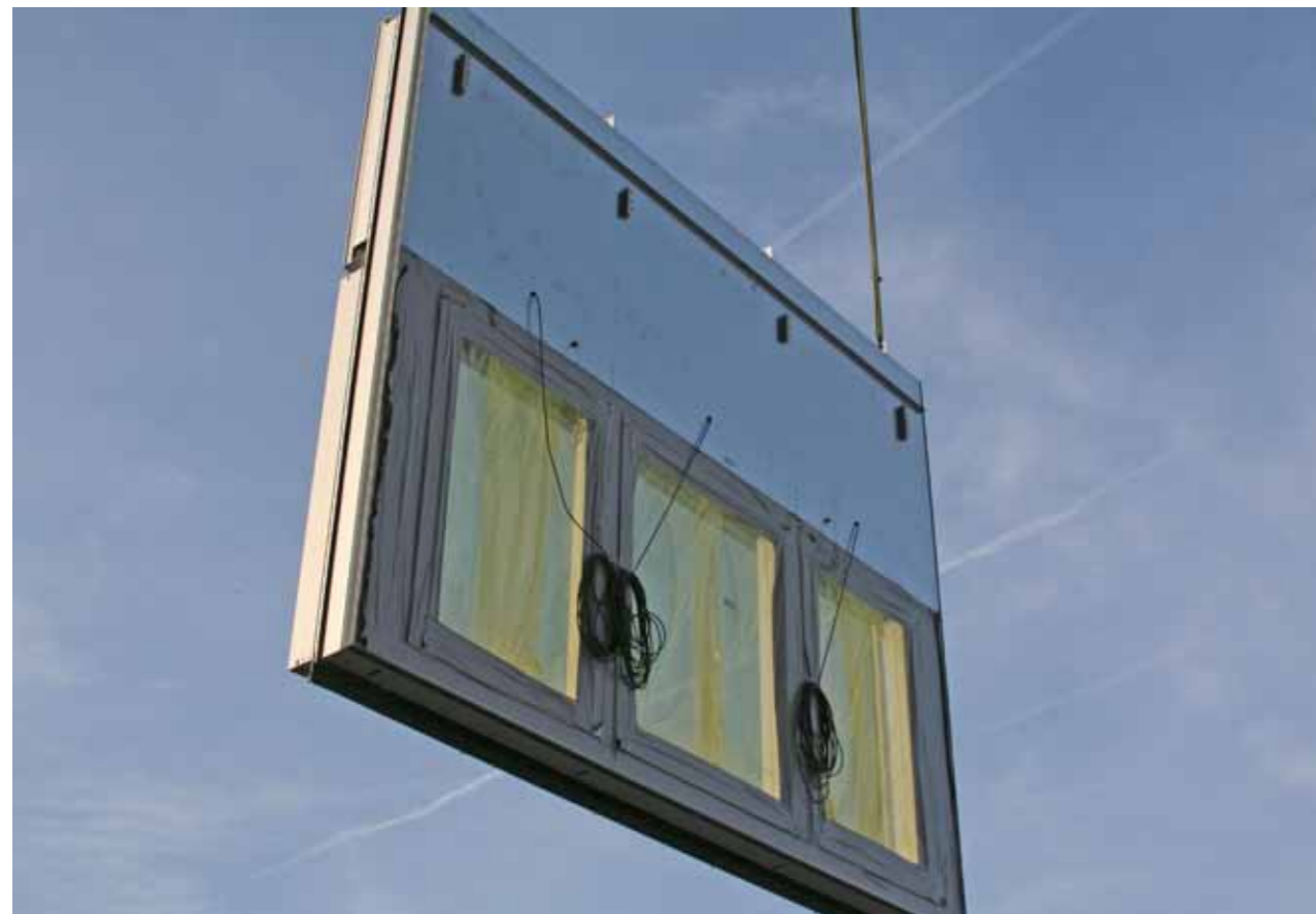
The new façade has a mechanical sun screen, which sits in the façade gap in front of the internal window façade and whose electric drive is also housed in the close-cavity façade.
